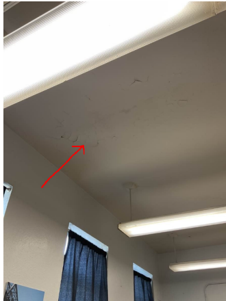
Multiple ceiling tiles and hard lid have water damage and should be repaired and replaced.
