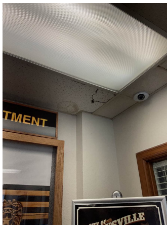
Multiple ceiling tiles and hard lid have water damage and should be repaired and replaced.
