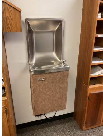
The hall drinking fountain shoots a high stream of water and needs to be replaced or adjusted.
