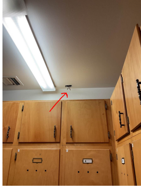
There are exposed wires and several lights out in the Men's locker room. Corridor plug seems to be damaged.
