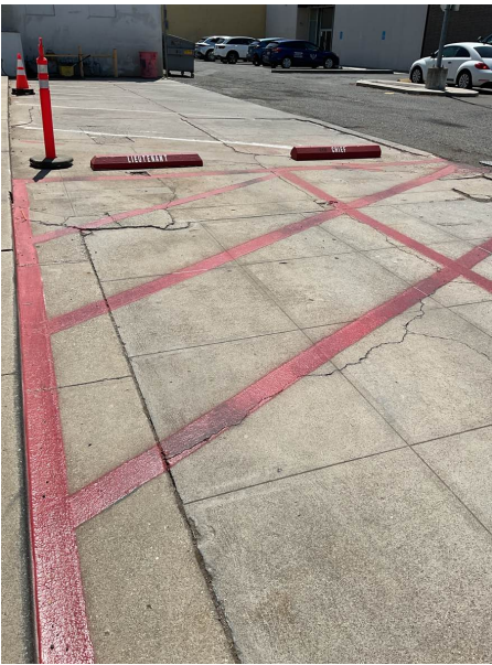
The entrance, sidewalk and private parking area have several large cracks and should be repaired.
