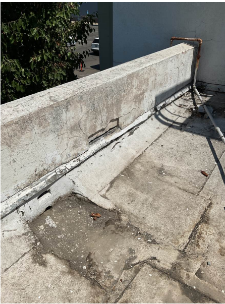
The roof flashings are damaged along parapet wall and need to be replaced.
